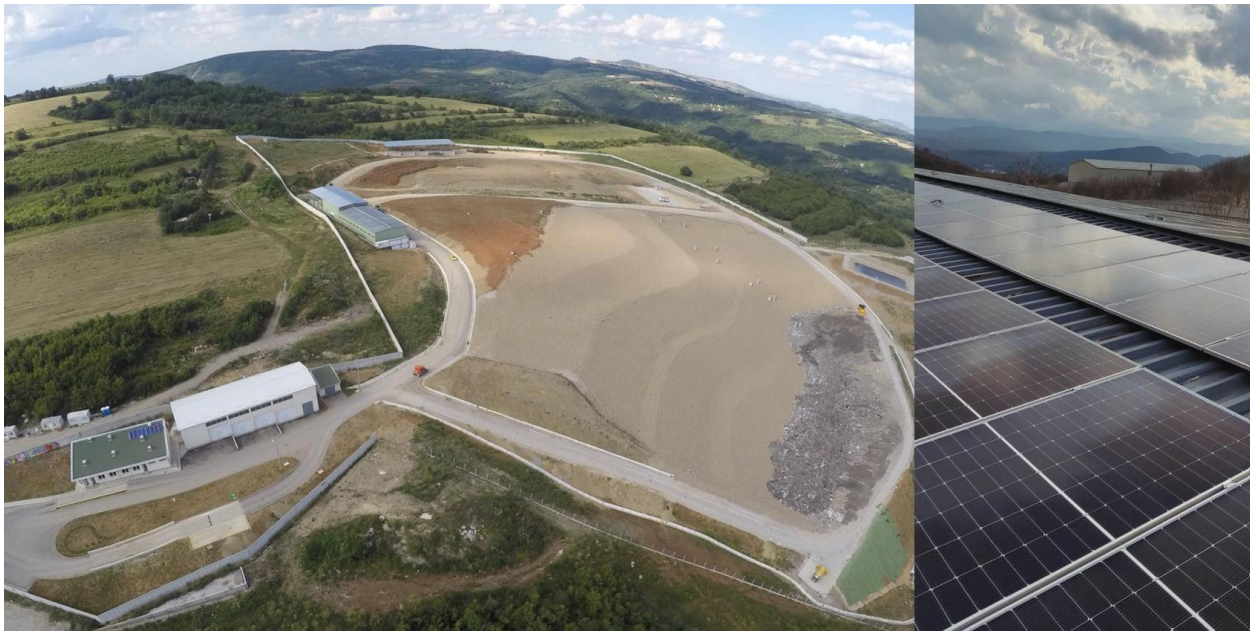
Figure 1 Aerial view of CEC Gabrovo
